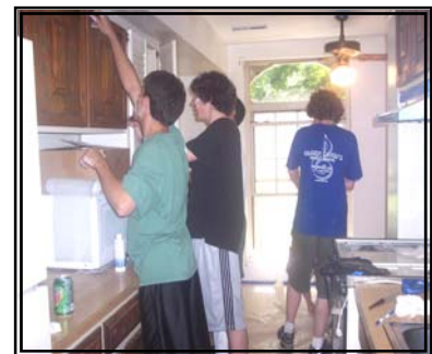
Scouts clean and paint the kitchen
